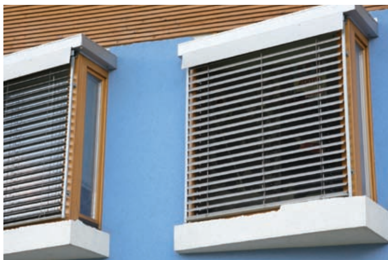
F-80 V (flat) alu vodila lamelle brez ojačanih robov
